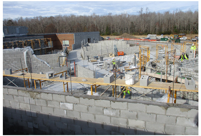
Hickory Middle School Building Addition Project
